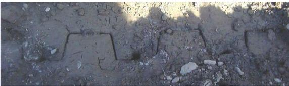
(b-3) Ground surface after pulled-out of sheet pile with chemical agent (Akaoka)
